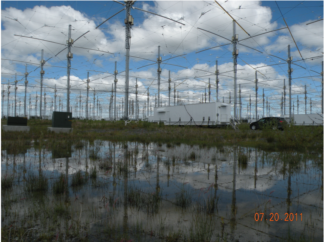
Figure 1-3. The HAARP HF heating facility. (Photo courtesy of Dr.Lee Synder.)
